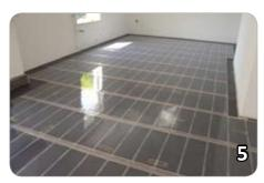
contact with or drop down onto the heating foil during the installation. Plan your work in a way that you don't have to step directly on the heating foil.
